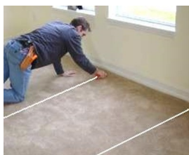
2. Cut or tear into manageable strips (around 3' wide 2 )
