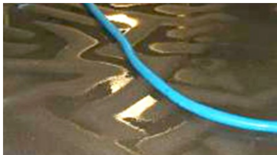
Carpet and pad now contain flood's contaminants
