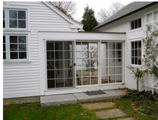
Closed in breezeway or patio - Yes (Mold spores can't escape to the open air, but will enter the residence)
