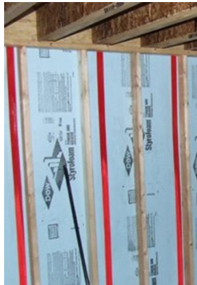
Closed cell Styrofoam
