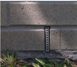
Metal vermin barrier
