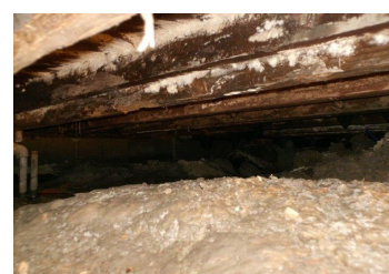
Dirt and debris restrict air flow
