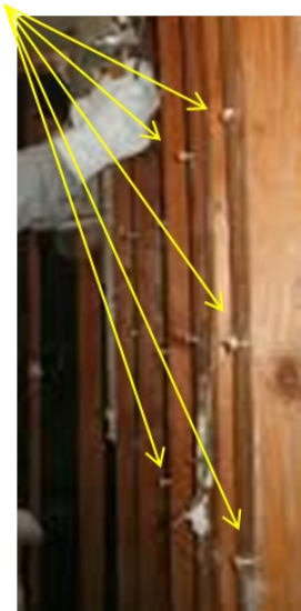
Pound in or pull out screws using hammer, claw or pry bar, or break screws by striking a glancing blow with hammer
