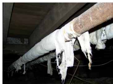
Hazardous asbestos insulation
