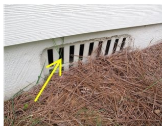
Vents plugged or non-existent
