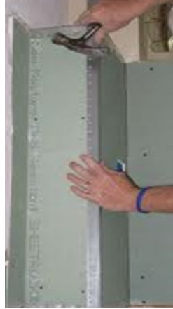
Hit corner bead a glancing blow to remove, or remove nails if nailed into place.
