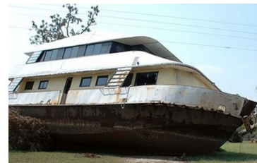
No - Structure is not in its dock and is unstable
