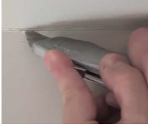
1. Cut drywall tape at the edge of removal area
