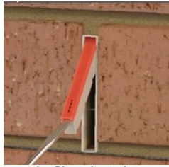
Air filter in joint
