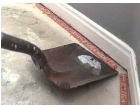
Remove tack strips with long handled shovel
