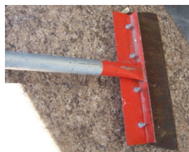
If the pad is glued down, use a floor scraper
