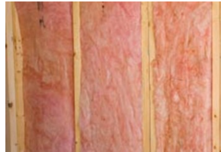
Fiberglass (itchy) - good chance of mold
