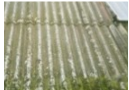
Cement roofing sheets and spray on sound proofing
