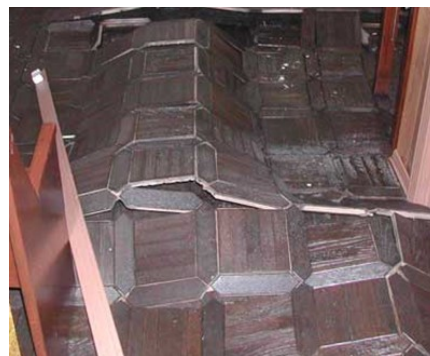
Floor damaged beyond repair
