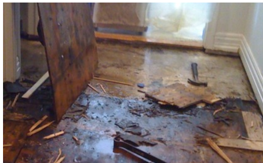
Water can't escape from multiple layered floors, causing mold growth if any layer is organic.
