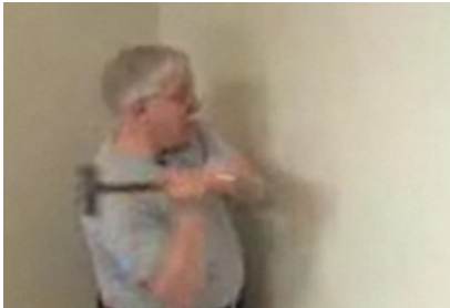
Make 2 hand holes, grab the rock and gently shake back and forth to remove large pieces
