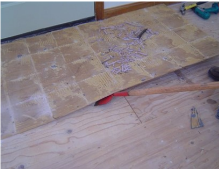
Remove tile by prying up backer board or plywood layer with tile scraper or flat shovel.
