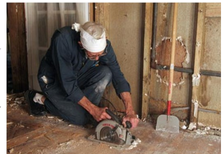
If cutting a floor, set saw depth so as not to cut floor joists
