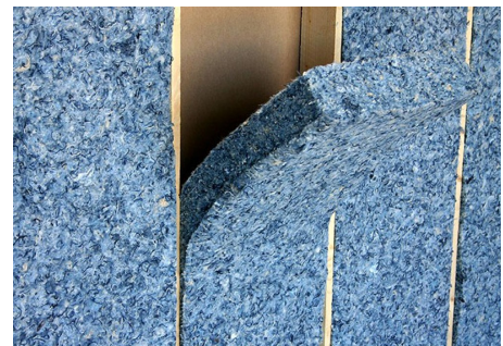
Denim fibers (not itchy) good chance of mold if water saturated
