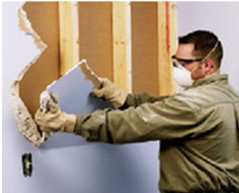
Make 2 hand holes, grab the rock and gently shake back and forth to remove large pieces
