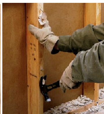
Pound in or pull out screws using hammer, claw or pry bar, or break screws by striking a glancing blow with hammer
