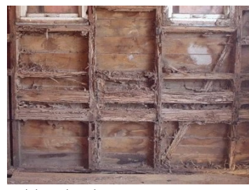
Termite damage can cause wall to collapse
